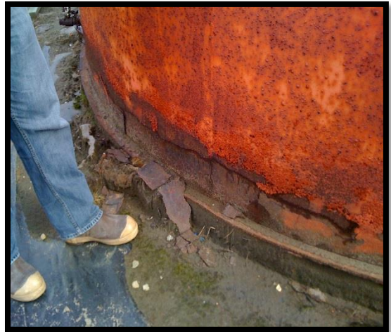
Tank Corrosion
