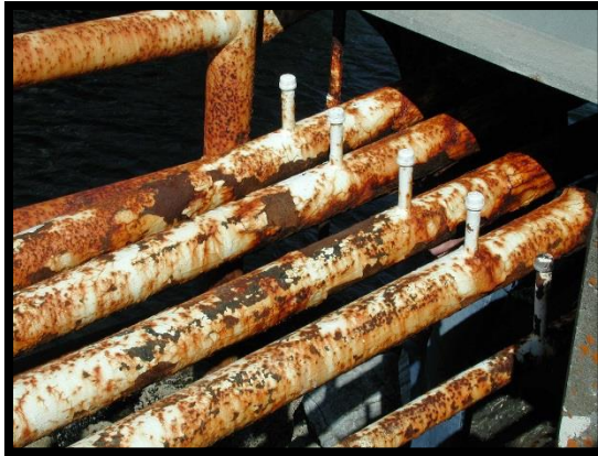
Pipe Corrosion
